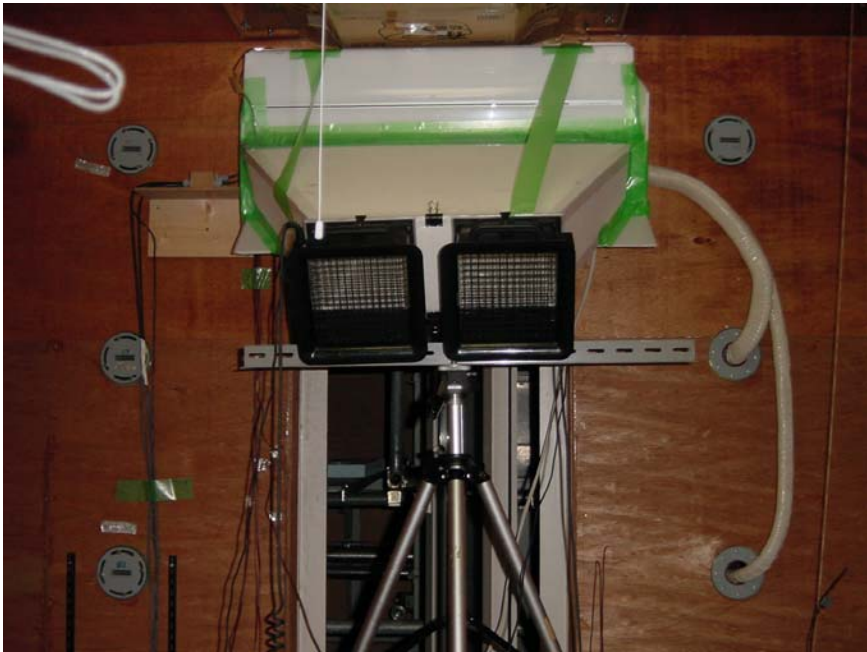
Measurement of Outlet Air Flow Rate
