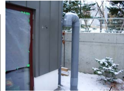
Heat and cool tube VP 200 mm \phi Depth=1.1m, Length=40m
