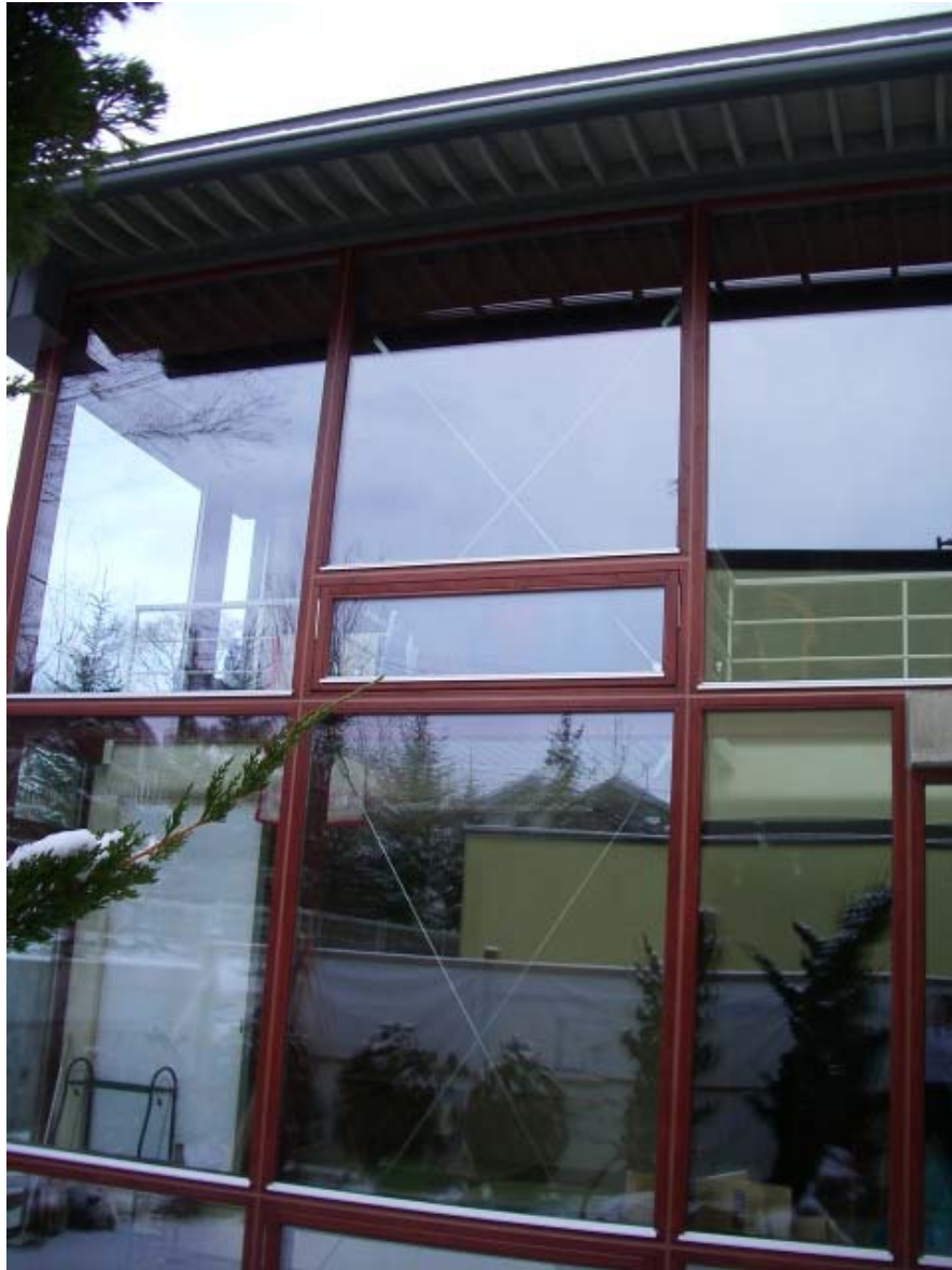
Southern glazing curtain wall construction
