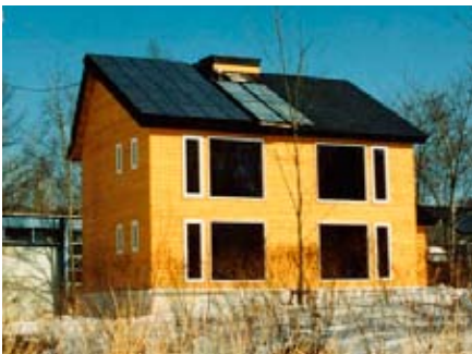
Photo 1 Low-energy experimental house at Hokkaido University
