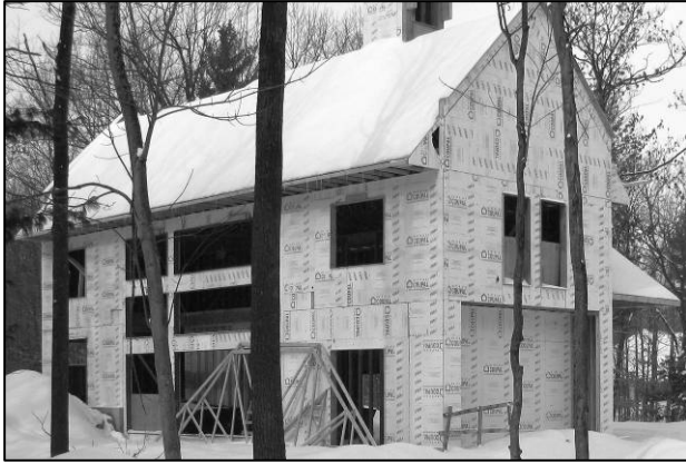
Figure 2. Alstonvale Net Zero House (under construction)
