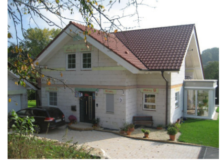
The front view of the monitored building
