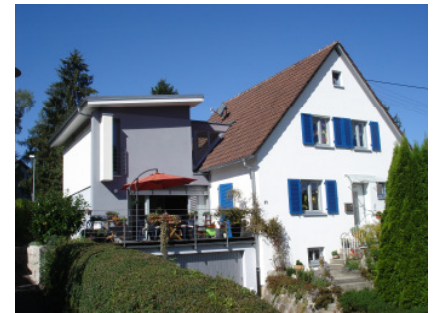
The front view of the monitored building
