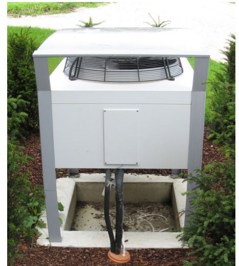
Evaporator of the split air-to-water heat pump unit
