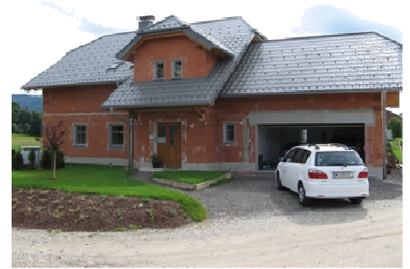
The front view of the monitored building
