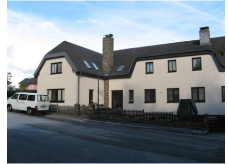
The front view of the monitored building
