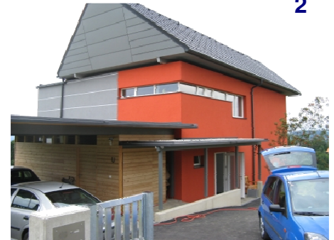
The front view of the passive house
